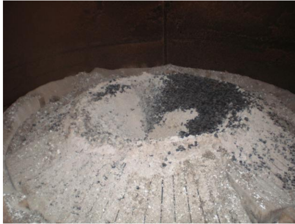
Ash chute inside furnace
