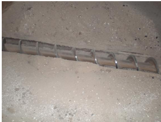
Ash Auger inside furnace
